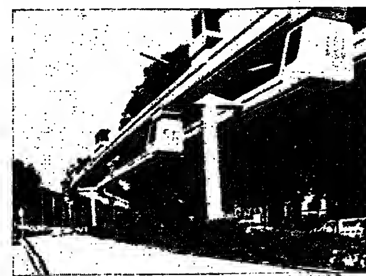
OVERHEAD RAIL—A montage of the proposed CAT system shows passenger cabins which would carry up to three persons at 20 miles an hour—twice as fast as streetcars go.
